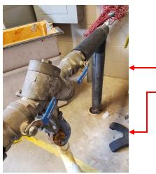
Turn the blue valves 90 degrees to shut off the water.
