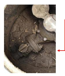
Remove the cover. Look for the valve. Insert the water key and turn 90 degrees.
