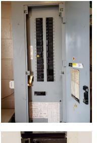
Open panel door. Look for breaker #40 (Sprinkler Control) near the bottom on the right-hand side.
