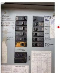
Locate the small electrical panel inside the enclosure under the gazebo. Open the panel door. Flip the corresponding breakers to the "ON" position.
