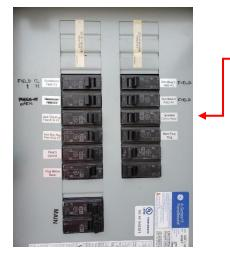
Look for the "Sprinkler Control" breaker and flip it to the right (or "off" position).
